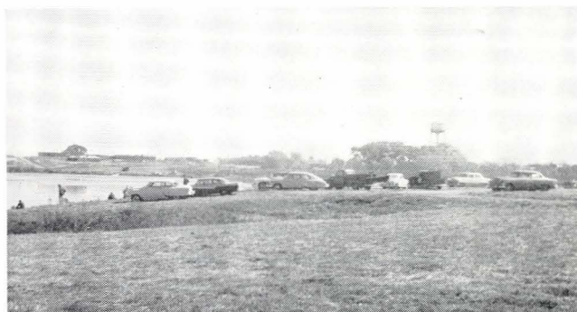
View of the dam at Barber County State Lake showing proximity to residential area of Medicine Lodge.
